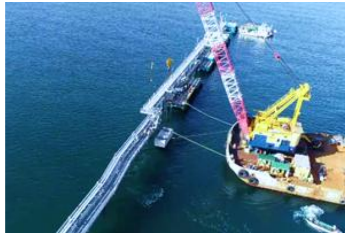
Rationalized Precast Pier Construction Method
