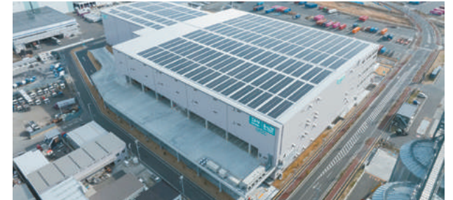
Nitori's ZEB-compliant Sendai Distribution Center
