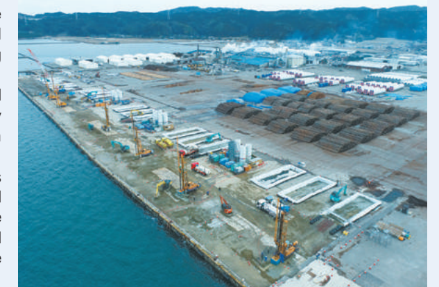
Disaster recovery work at Ota Quay, Port of Nanao
