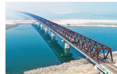
► Jamuna Railway Bridge Construction, Eastern Part of Civil Works Package WD1* Client: Ministry of Railways, People's Republic of Bangladesh
