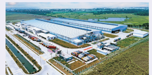
Environmentally conscious production facility of Singer Bangladesh Limited constructed by TOA CORPORATION
