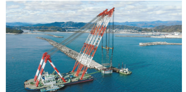
Breakwater construction work at Kochi Port
