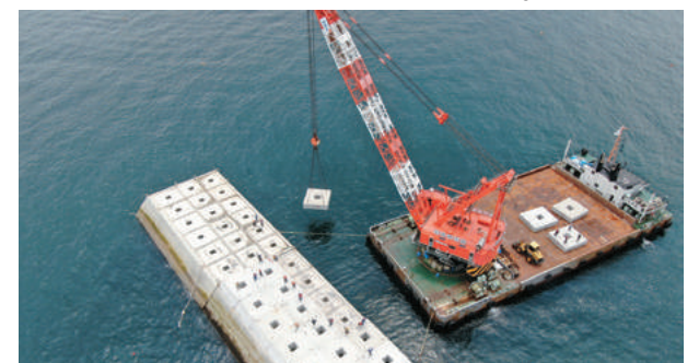
Precast superstructure installation in progress
