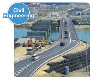
▲ Kesen Ohashi Temporary Bridge Construction
