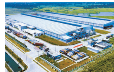
► Singer Bangladesh Home Appliances Plant Construction (Package-2) Client: Singer Bangladesh Limited
