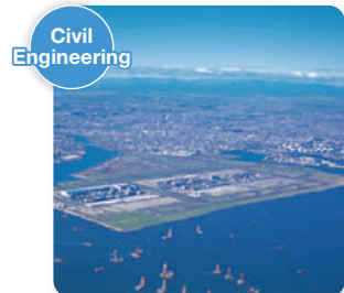
▲ Haneda Airport Re-Expansion Project
