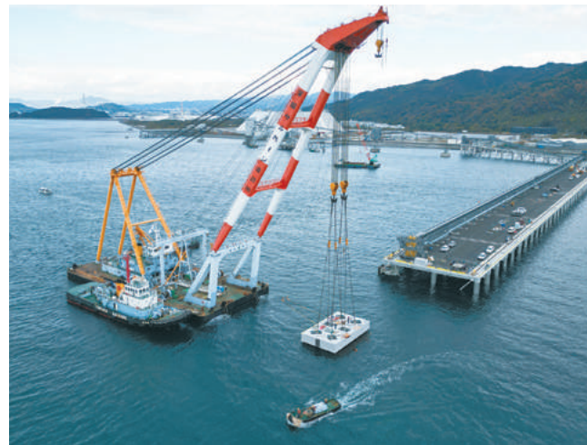
Precast superstructure installation
