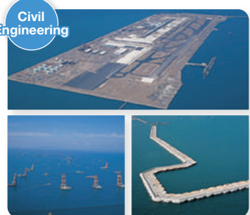
▲ Kansai International Airport Phase 1 Construction
