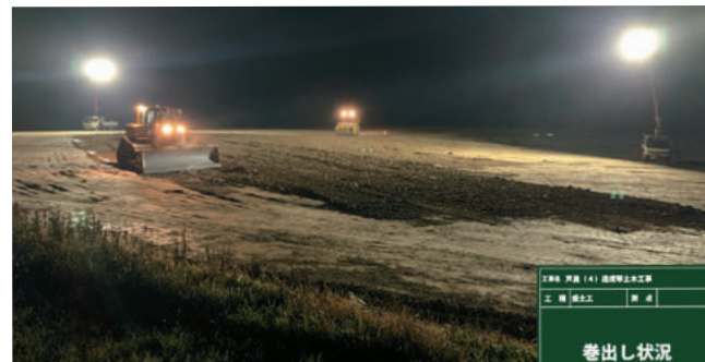
Embankment leveling using ICT-equipped machinery
