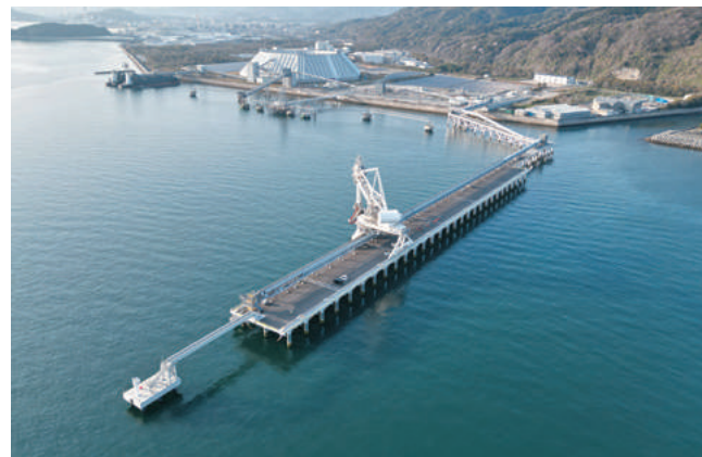
Completed pier (~19 m) at Tokuyama-Kudamatsu Port, Kudamatsu District
