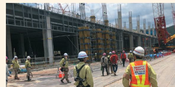
▶ Joint patrols at worksites
