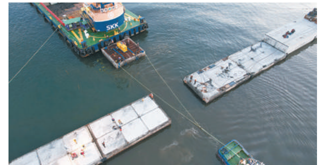
Caisson installation work
