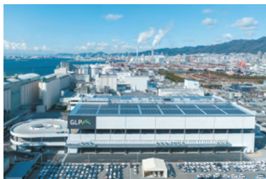
► GLP Kobe Sumiyoshihama Project (tentative name) Client: GLP Kobe Sumiyoshihama Special Purpose Company
