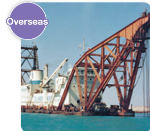
▲ Arab Republic of Egypt Dredging Work at Suez Canal
