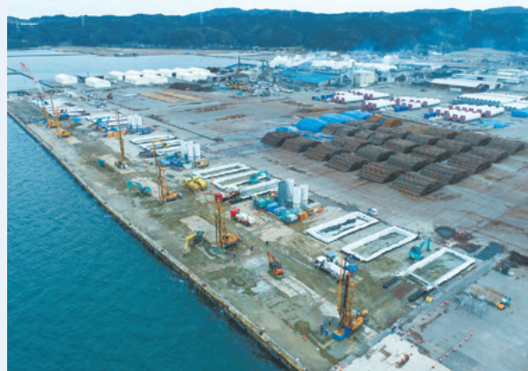
Disaster recovery work at Ota Quay, Port of Nanao
