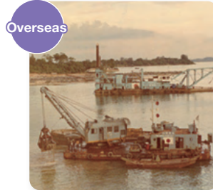
▲ Republic of Singapore Dredging Work at Jurong Islands
