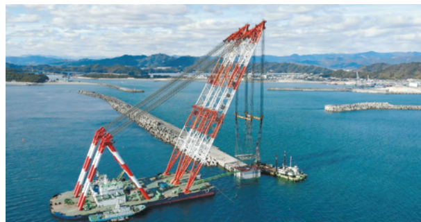
Breakwater construction work at Kochi Port
