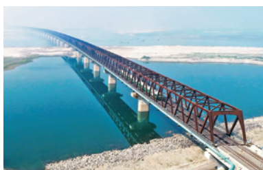
► Jamuna Railway Bridge Construction, Eastern Part of Civil Works Package WD1*
