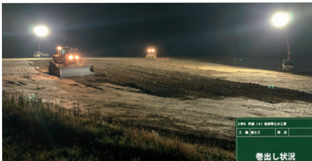
Embankment leveling using ICT-equipped machinery
