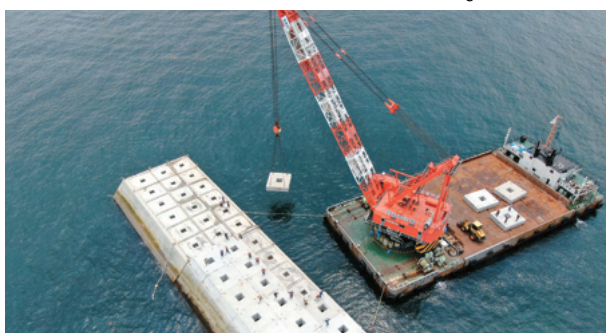
Precast superstructure installation in progress
