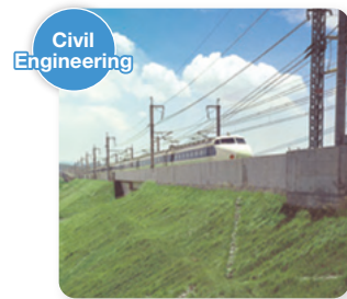
▲ Sanyo Shinkansen Nishi-Asa District Construction
