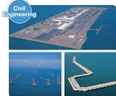
▲ Kansai International Airport Phase 1 Construction
