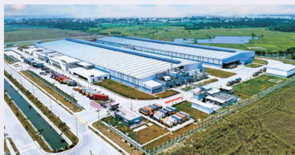
Environmentally conscious production facility of Singer Bangladesh Limited constructed by TOA CORPORATION
