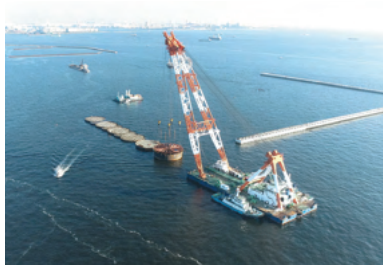
► FY2023: Construction of Shin-Honmoku Pier (-18 m, seismic) at Port of Yokohama (Phase 2)
