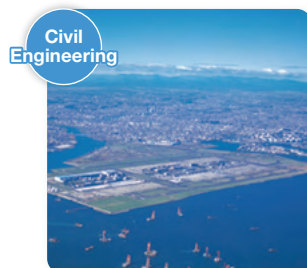
▲ Haneda Airport Re-Expansion Project
