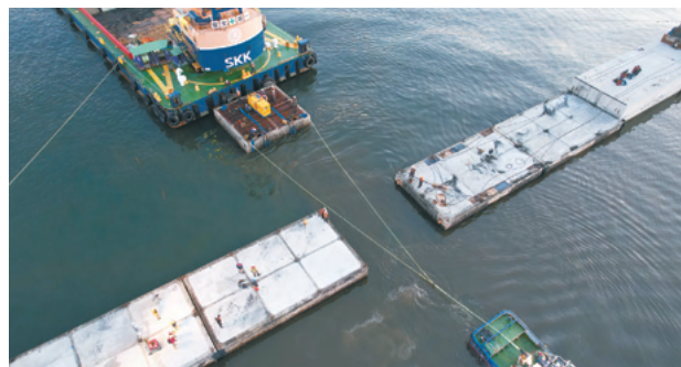
Caisson installation work
