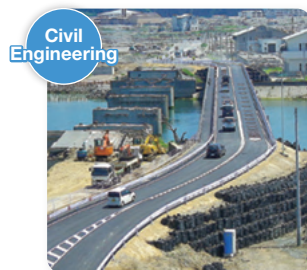
▲ Kesen Ohashi Temporary Bridge Construction
