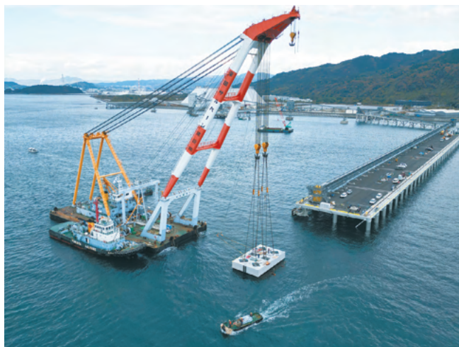
Precast superstructure installation
