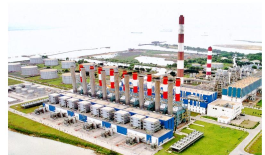
Gresik Power Plant (Civil Works) Indonesia (1994)
