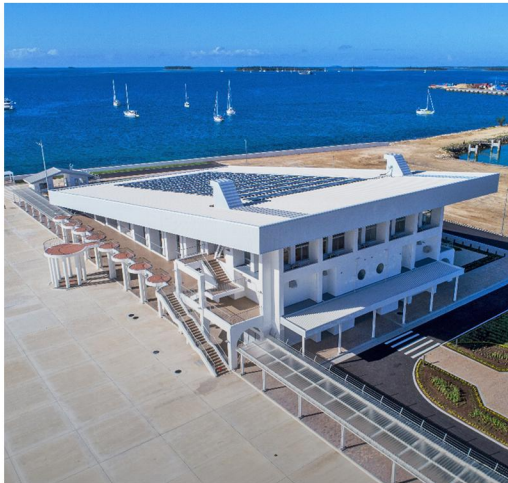
Passenger Terminal at Fuaa Wharf (3-storey; est. 2,900sqm.)
