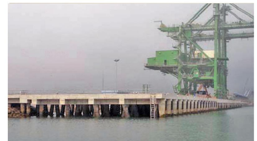
Nghi Son 1 Power Plant (Jetty Works) Vietnam (2013)
