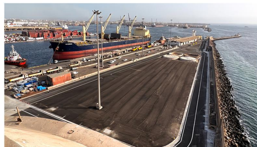
Third Wharf in Dakar Port Senegal (2022)
