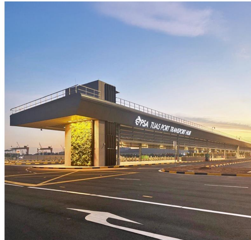
Tuas Port Transport Hub (Sheltered boarding and alighting areas for public buses)
