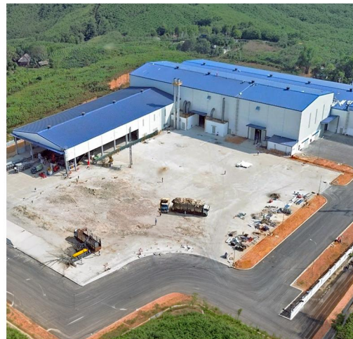
EREX Sakura Pellet Factory (Steel Structure; est. 21,000sqm.) Country: VIETNAM (2025) Client: EREX Sakura Biomass Tuyen Quang Co., Ltd.
