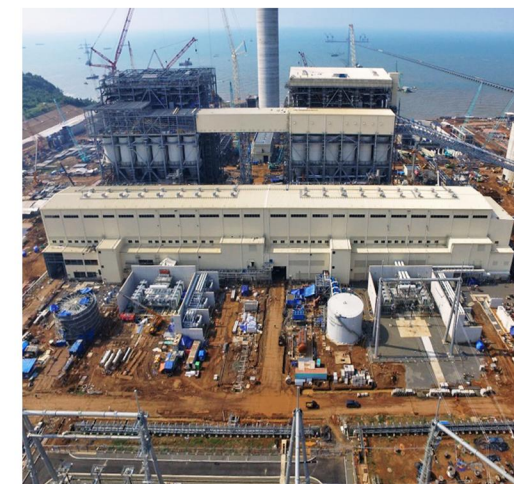
Central Java Coal Fired Power Plant (2x1000 MW) [Turbine building construction]
