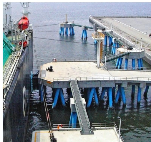
Northern LNG Receiving Terminal [Dolphin-type berth construction & dredging works]
