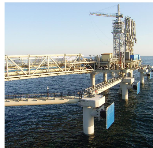
Sakhalin II LNG Terminal [Approach trestle & dolphin-type berth construction]
