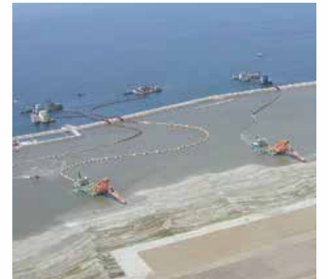
TOA's "Plug Magic" dredging method was adopted in order to maximize the recycling of dredged soft materials
