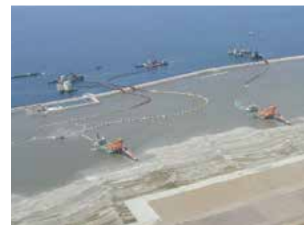
TOA's "Plug Magic" dredging method was adopted in order to maximize the recycling of dredged soft materials
