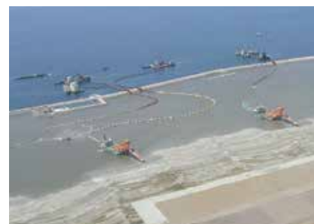
TOA's "Plug Magic" dredging method was adopted in order to maximize the recycling of dredged soft materials
