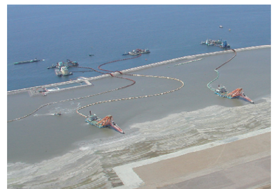
TOA's "Plug Magic" dredging method was adopted in order to maximize the recycling of dredged soft materials
