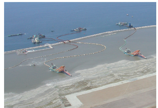
TOA's "Plug Magic" dredging method was adopted in order to maximize the recycling of dredged soft materials
