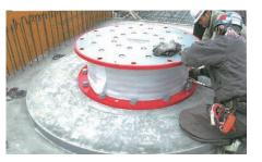
A construction method where layered rubber is inserted in between the building and foundation and by separating the foundation from the building, the sharp movements of an earthquake are changed into slower, more gradual movements. This maintains the safety of the people inside the building and protects the building and equipment from damage. FRP Protective Permanent Form Method -Salt Damage Deterioration Restoration-
