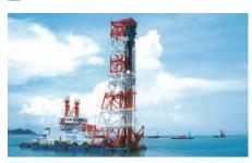
A Cement Deep Mixing method. This method hardens soft foundations by mixing soft soil with a stabilization agent in-situ using a rotating mixing shaft with blades. The method is suitable for providing stable strength quickly in both onshore and offshore works and for various purposes such as massive constructions, narrow space construction and treatment of contaminated soil.
