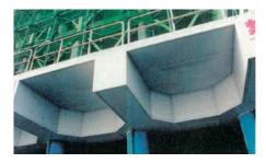
A restoration method for concrete port structures suffering from salt damage. Highly rigid FRP\* panels are used as a framework when restoring the deteriorated parts, and the panels are left in place after completion of the work to prevent penetration of external chloride ions, making for a durable structure. \*FRP: Fiber Reinforced Plastics
