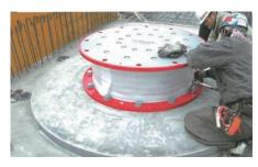
A construction method where layered rubber is inserted in between the building and foundation and by separating the foundation from the building, the sharp movements of an earthquake are changed into slower, more gradual movements. This maintains the safety of the people inside the building and protects the building and equipment from damage.
