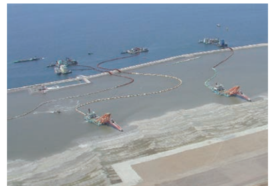
TOA's "Plug Magic" dredging method was adopted in order to maximize the recycling of dredged soft materials
