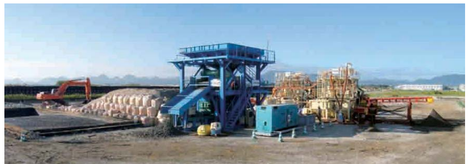
A panoramic view of the facilities
