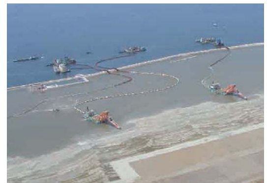
TOA's "Plug Magic" dredging method (see page 14 for details) was adopted in order to maximize the recycling of dredged soft materials
