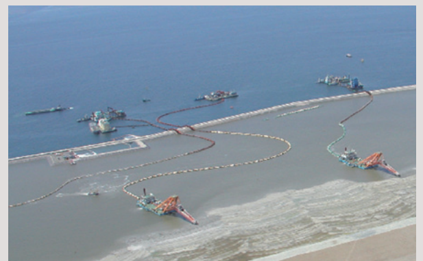
TOA's "Plug Magic" dredging method (see page 12 for details) was adopted in order to maximize the recycling of dredged soft materials
