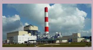
O Mon Thermal Power Plant with 330MW generation capacity in Can Tho, the biggest city in the Mekong Delta, was planned to solve the growing shortage in electric supply in Vietnam. Under the full turn-key contractor of the project, TOA took charge of all civil and architectural works, and completed them in 2009. TOA's expertise in geotechnical engineering was especially evaluated as the soft alluvial clay layers lying under the plant site had to be improved to construct solid foundations on them.
