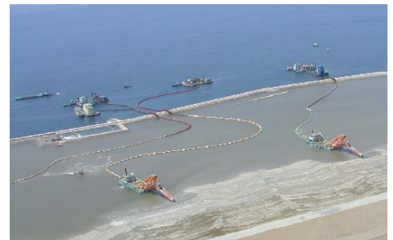
TOA's dredging method "Plug Magic" (see page 12 for detail) was adopted in order to maximize the recycle of dredged soft materials.
