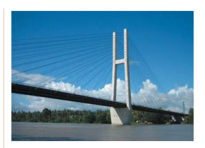
Toa Corporation completed the construction of the bypass road extending 8100m, two installation roads extending 1330m and 1640m, a steel-made cable stayed bridge of 360m in length, elevated bridges for approaching the main bridge which extends 372m to the east
