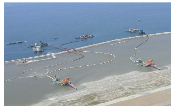
TOA's dredging method "Plug Magic" (see page 12 for detail) was adopted in order to maximize the recycle of dredged soft soil.
