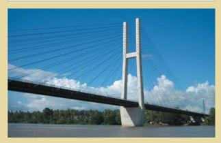
Toa Corporation completed the construction of the bypass road extending 8100 meters, two installation roads extending 1330 meters and 1640 meters, a steel-made cable stayed bridge of 360 meters in length, elevated bridges for approaching the main bridge which are extending 372 meters to the east and 150 meters to the west, and their related facilities.
