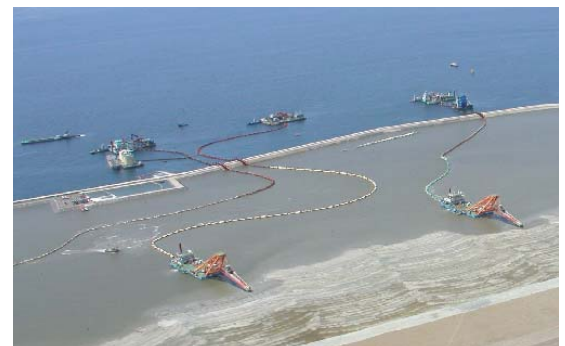
TOA's dredging method "Plug Magic" (see page 12 for detail) was adopted in order to maximize the recycle of dredged soft soil.
